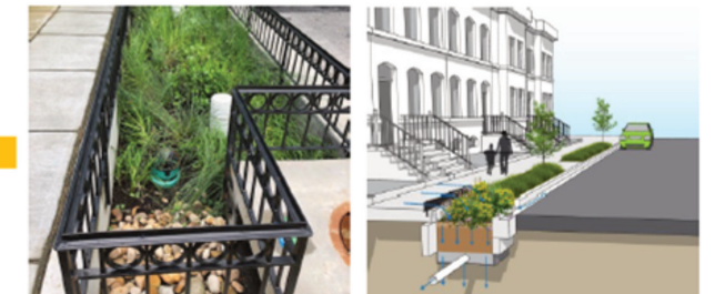
Planter Bioretention (PBR)
