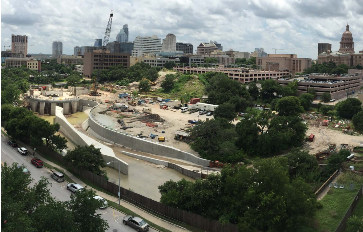
Bypass Tunnel Infrastructure
