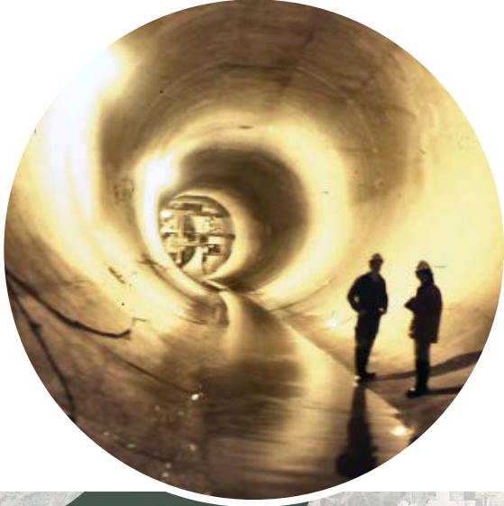
26-ft diameter tunnel ~70 ft below the surface
