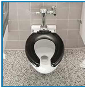
Flushometer Valve Toilets
