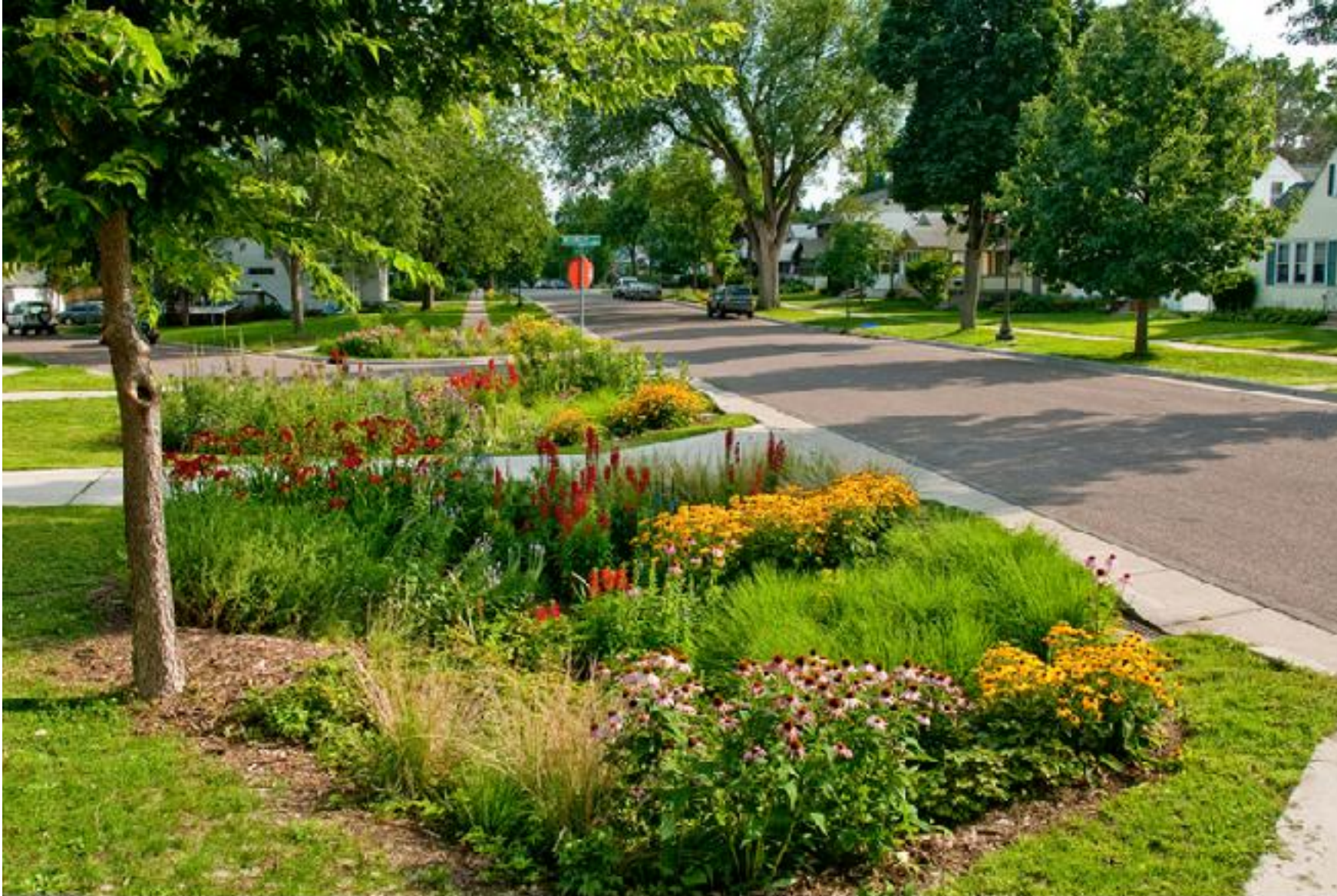
This rain garden is taking advantage of a low area of the yard, slowing and reducing the amount of runoff that reaches the storm drain. Photo: Capitol Region Water District.
