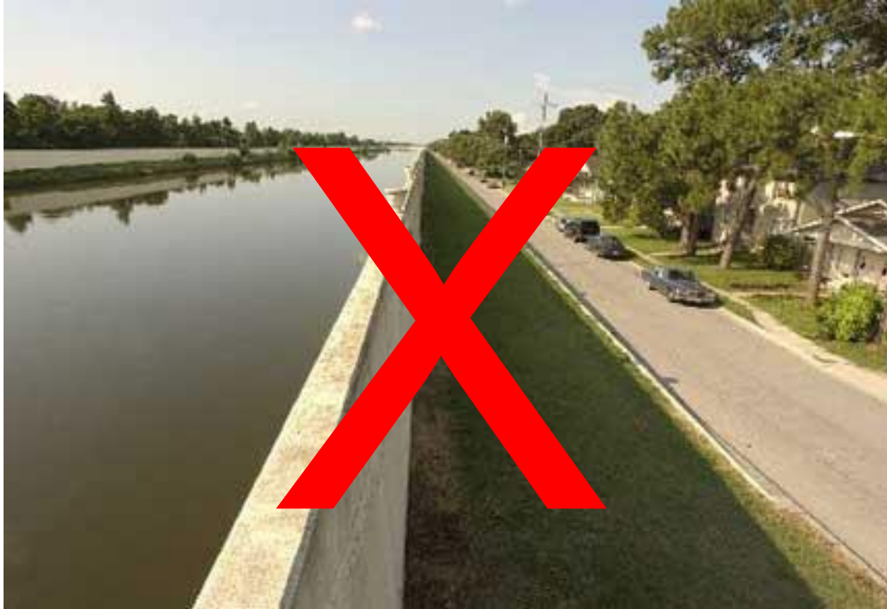
New Orleans floodwall
