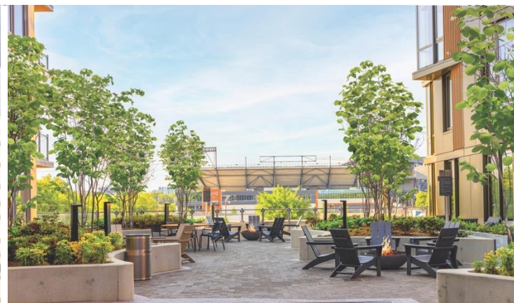
River Point | LEED Gold | Photo: Ray Cavacchio
