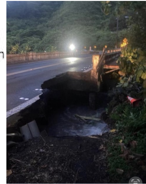
Kahana Bridge July 16, 2022
