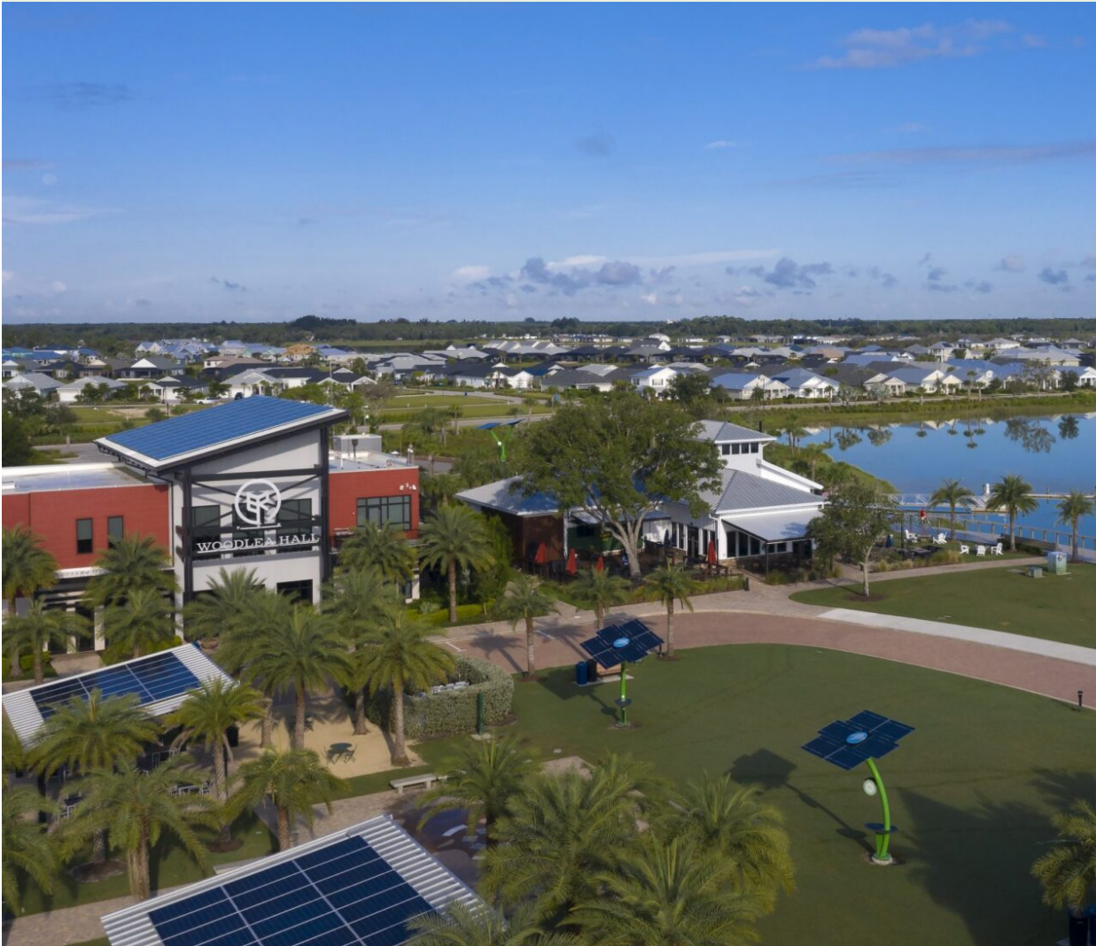
FIGURE 29 Drone photo of Babcock Ranch community facilities and solar arrays. ( Babcock Ranch )
