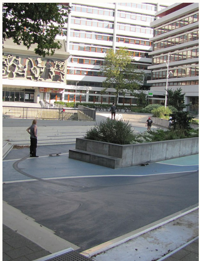
Bentheimplein Water Square in Rotterdam acts as a multipurpose rainwater collection basin during floods as well as a recreational space.
