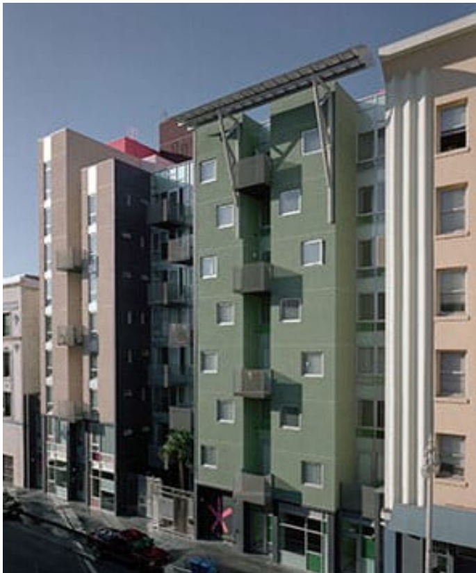
In place of parking in San Francisco, Curran House's ground floor includes community spaces, a peaceful courtyard, office space for the building developer, and additional affordable family-sized units. (Brian Rose)
