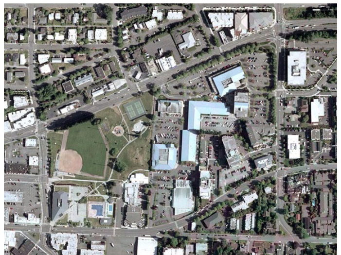
The original Parkplace Center, an 11.5-acre (4.7 ha) strip center, was built in 1980 and anchored by a 25,000-square-foot (2,300 sq m) QFC grocery. (CollinsWoerman)
