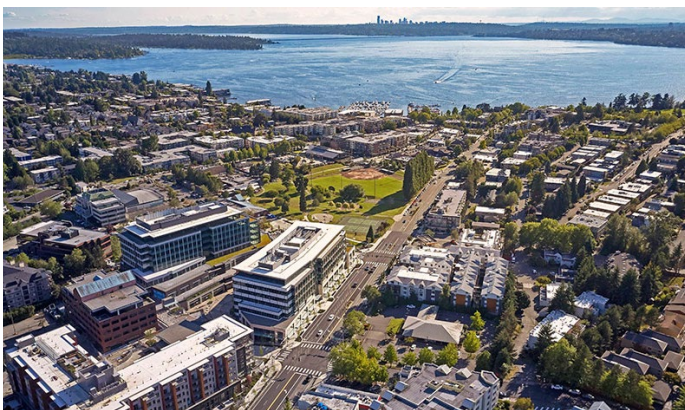
The recent state of completion of Kirkland Urban. The red-brick Parkland Place office building has not yet been replaced by Kirkland East. (CollinsWoerman)
