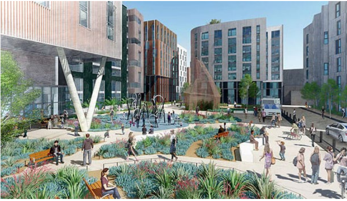
The Brady Block, in design in San Francisco, will have 600 new units of housing, a new office building, a new public realm, and streetscape improvements on Market Street—plus a 0.5:1 parking ratio. (David Baker Architects)
