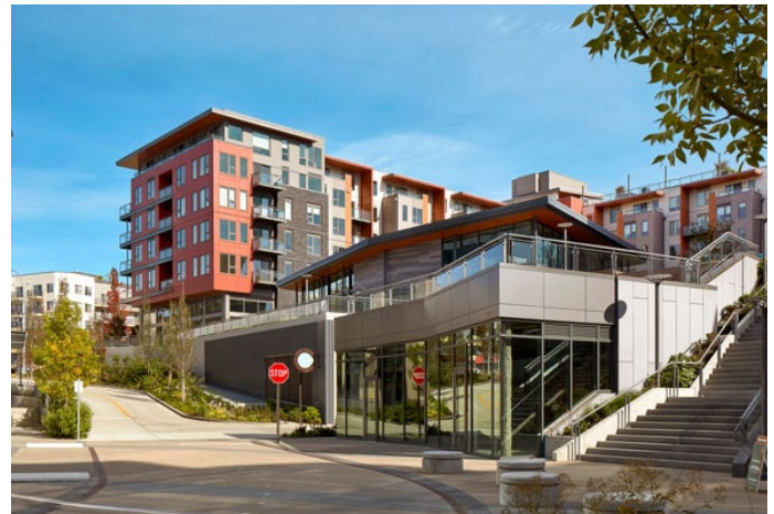
The slope of the site, which descends more than 35 feet (11 m) from east to west, allowed architects to bury the bulk of the blank walls of the grocery store, loading docks, and cinemas in the slope.
