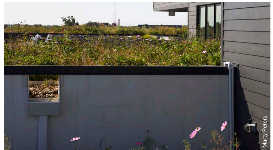
At District House, lawned terraces on one floor of the multifamily building and a rooftop wildflower meadow resulted in a building that connects tenants to nature, while providing the developer with a strong return on investment.
