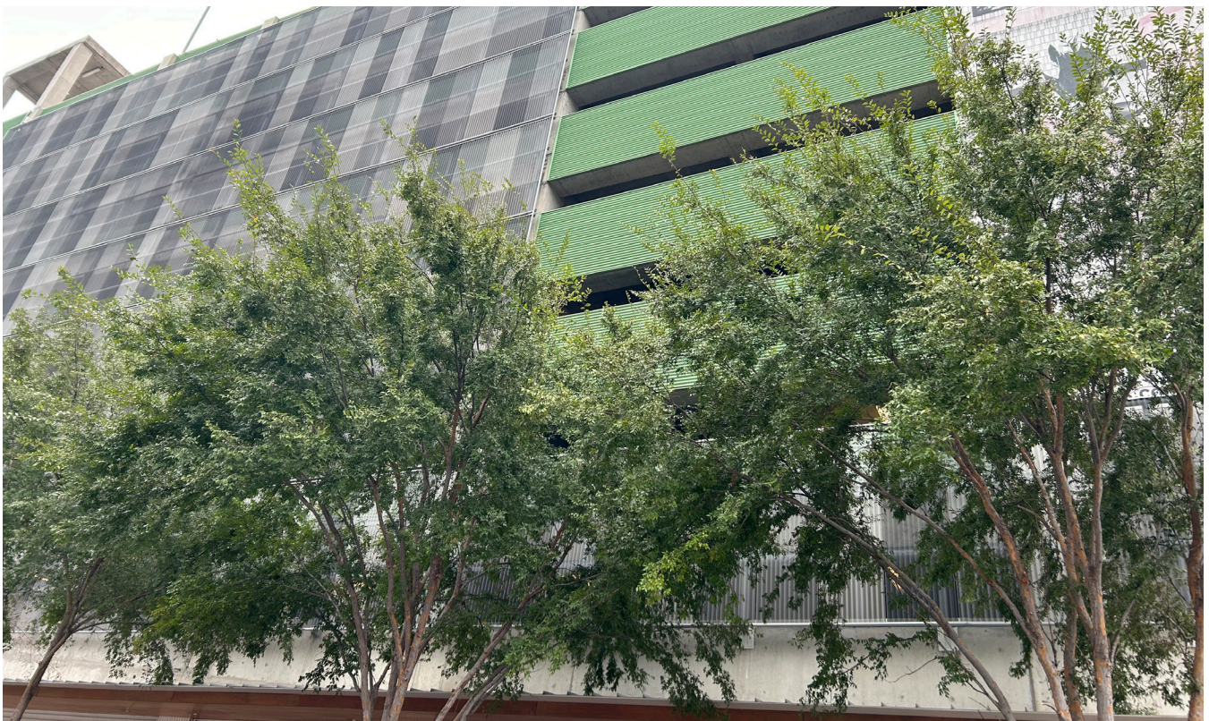
Screens and other architectural treatments can help to hide layers of parked cars but the lack of engagement with the street remains.
