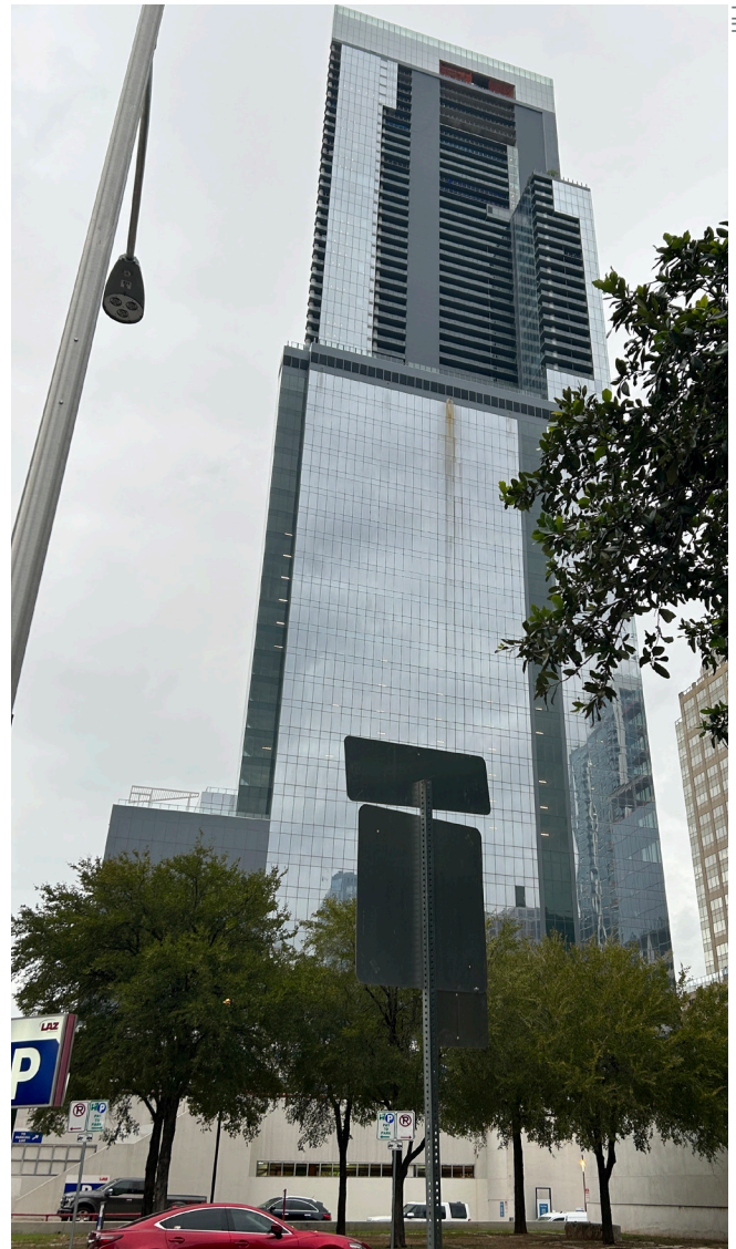
New development in downtown Austin still incorporates multiple levels of garage parking for tenants.
