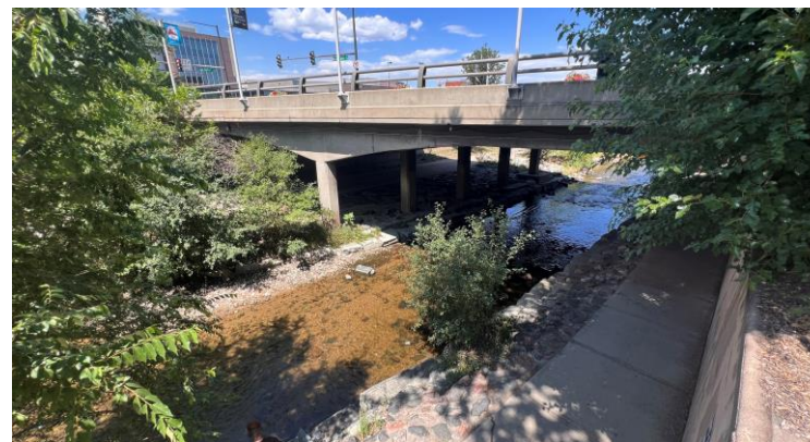
Lack of activating uses/destinations
