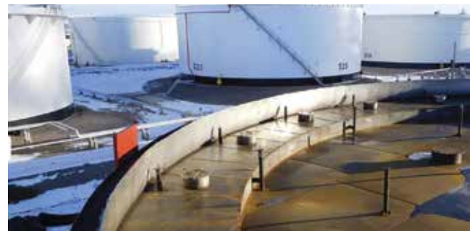
Several existing industrial businesses such as Epic Metals and Phillips Tank and Structure represent the traditional manufacturing that is thriving in EastShore.
